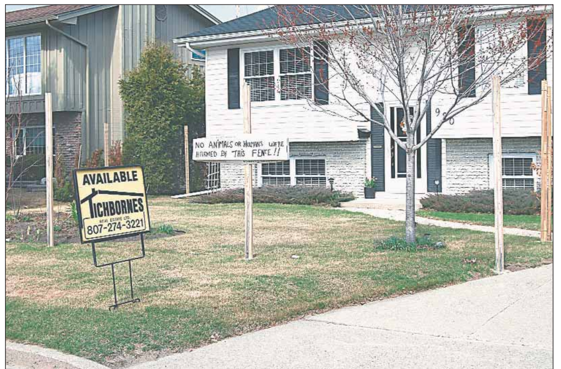
The picture above shows the fence that caused all the trouble. The trouble is, you can't see it because it is quite invisible.
