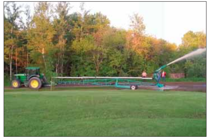
The Herman Krahn family from Dawson Twp. arrived to help and brought their manure spreader which was an efficient way to quickly move water from one side of the road to the river on the other. They saved the day in several locations in Rainy River.
