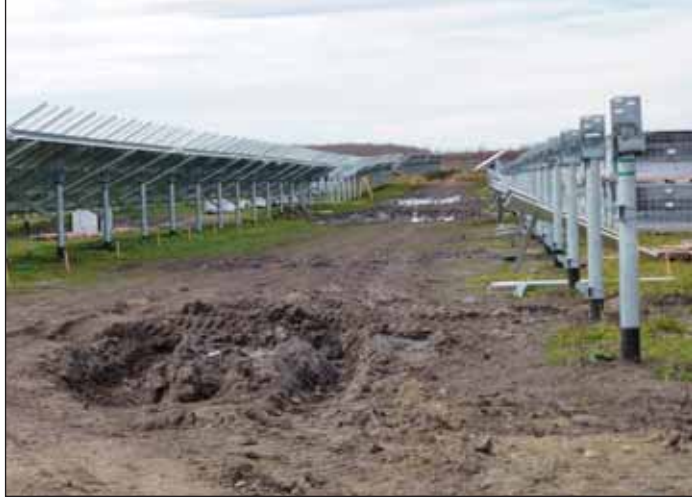
Pilings, or screws, waiting panels, beside a road before gravel was used. It was easy to understand, after seeing this, why there have been gravel trucks going into the sites all summer.
