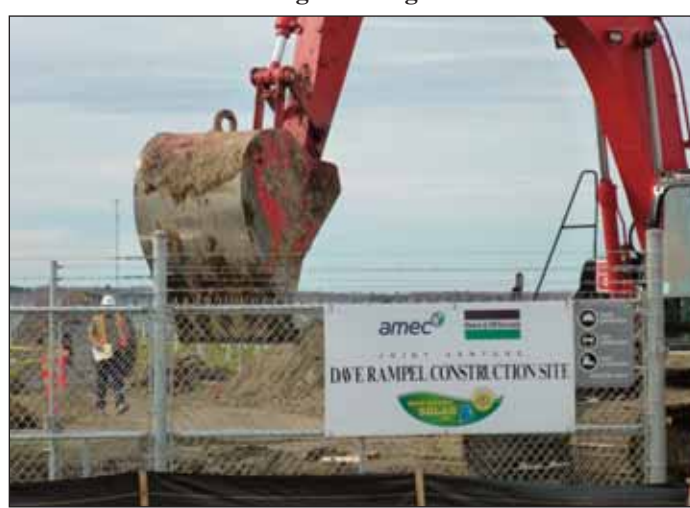
No equipment is moved or other heavy work done until a safety report is designed by Glen Lagacé, the Safety Manager. If needed a design is drawn up. When the report is complete, the work to be done is checked by a member of the safety team. Worker safety is taken very seriously by Black & MacDonald.
