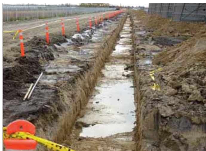
Trenches are dug between the pilings. The panels connect to wires which travel along a trough to collector panels situated between the rows of panels. These then connect to cables that are laid into the troughs ending at the vault.
